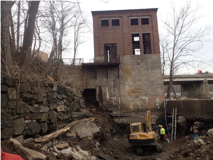
The Collinsville powerhouse will be re-used. A cofferdam was set at the end of the tailrace, which was de-watered so they could dig out accumulated sediment. The lower portion of the future fishway will emerge from the dark hole to the left and cross below the powerhouse and the entrance will be off photo to the right.
