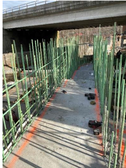
The footing/floor of the upper fishway is poured and this shows the walls being formed. Those walls have been poured by now. The upper fishway will pass under the Rt. 179 bridge.
